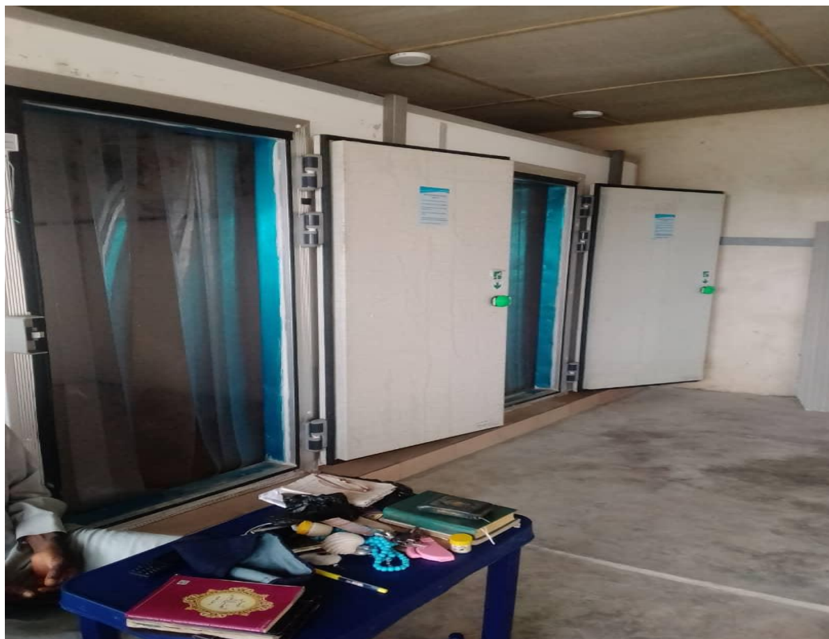
Fig 4: The cold room and the blast freezer
